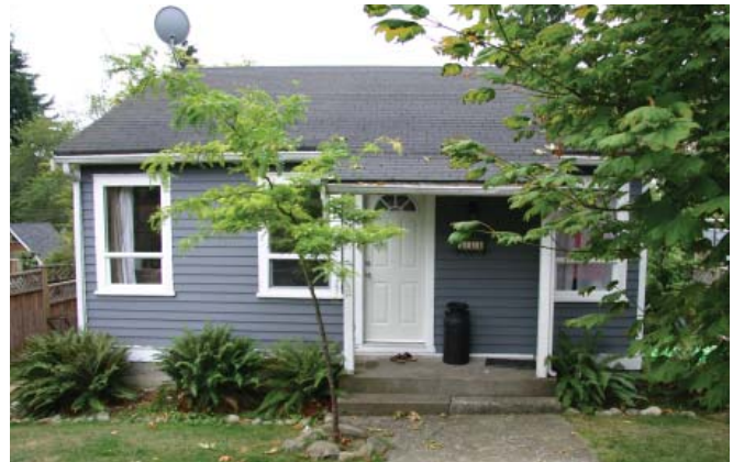
RUSHEDE RESIDENCE (Wartime Housing Ltd.) 733 East 3rd Street McCarter & Nairne, Architects 1941 REGISTER RANKING: A
