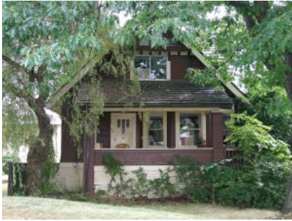
LAWRENCE RESIDENCE 423 East 6th Street 1908 REGISTER RANKING: B
