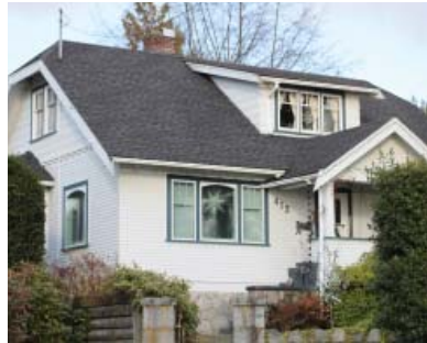
BENNETT RESIDENCE 412 East 5th Street 1928 REGISTER RANKING: B
