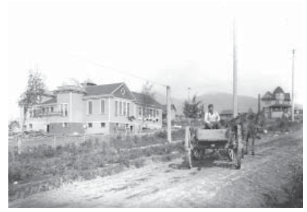
CENTRAL SCHOOL 333 Chesterfield Avenue/ 209 West 4th Street circa 1902; Major Additions 1907 REGISTER RANKING: A
