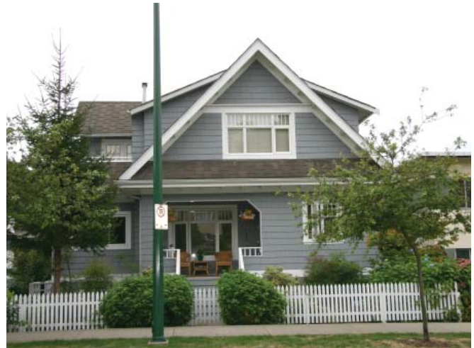
WHEELER HOUSE 155 East 4th Street 1914 REGISTER RANKING: B
