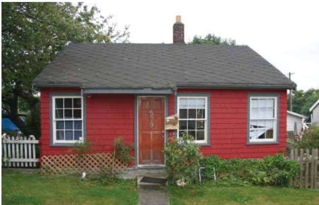
EATHERINGTON RESIDENCE (Wartime Housing Ltd.) 529 East 3rd Street McCarter & Nairne, Architects 1941 REGISTER RANKING: A
